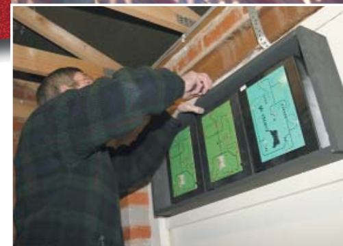
Upgrading an existing system.
