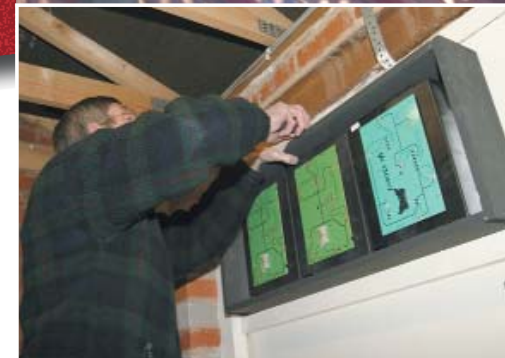
Upgrading an existing system.
